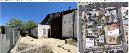
The original 1915 Teatro Carmen stagehouse & stage was removed in 1936 by the then-owners, the Black Elks Club. We are rebuilding those elements as part of the second phase of the project, which entails replacing the unsafe roof of the Theatre space with new trusses and decking along with the stage house rehabilitation. While we will not install the final theatrical equipment at this stage, we will be doing all of the infrastructure for the eventual lighting, sound, and film presentations.
