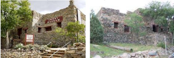
Funds will be used to stabilize and rehab the two historic buildings built in the 1930s, largely by hand, using local river stone and raw timber. The Museum and the Pueblo buildings' exterior rock walls require immediate attention; tuck pointing mortar joints and applying exterior sealant; patching and sealing both leaking roofs; crafting and replacing the Pueblo's twelve custom windows and all 57 exterior architectural viga tails. The project cost includes labor and materials.
