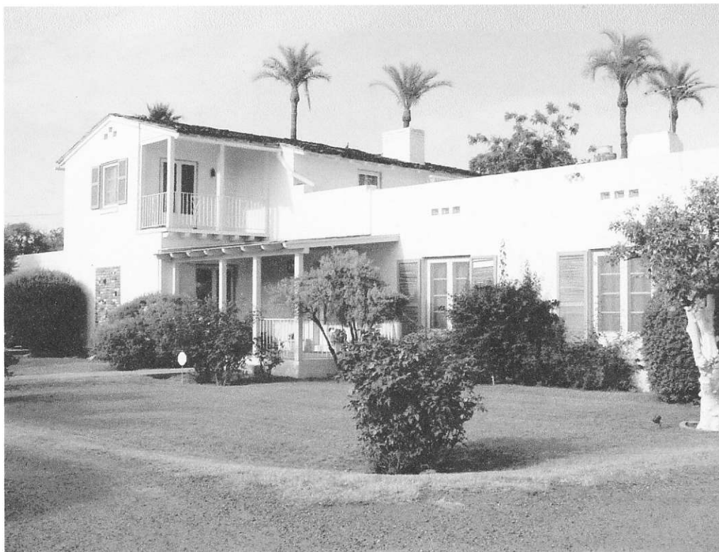
Figure 18. Col. Edward Power Conway House.
