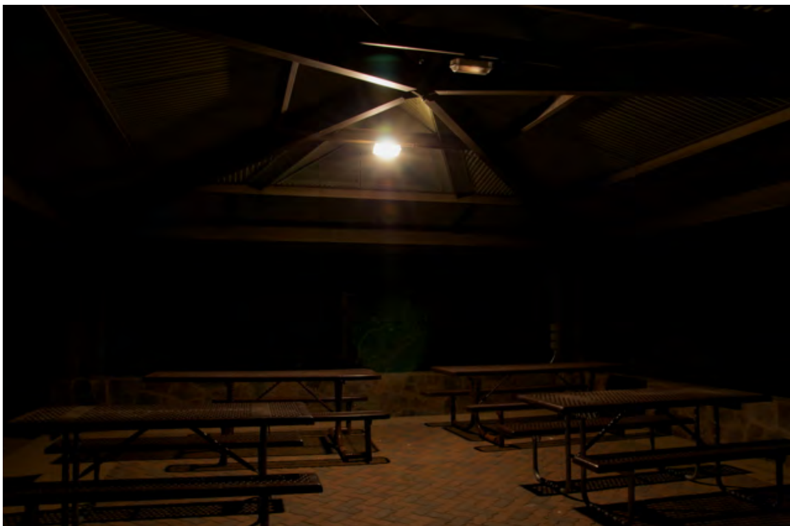
Figure 6.7 Group Use Area shelter lights
