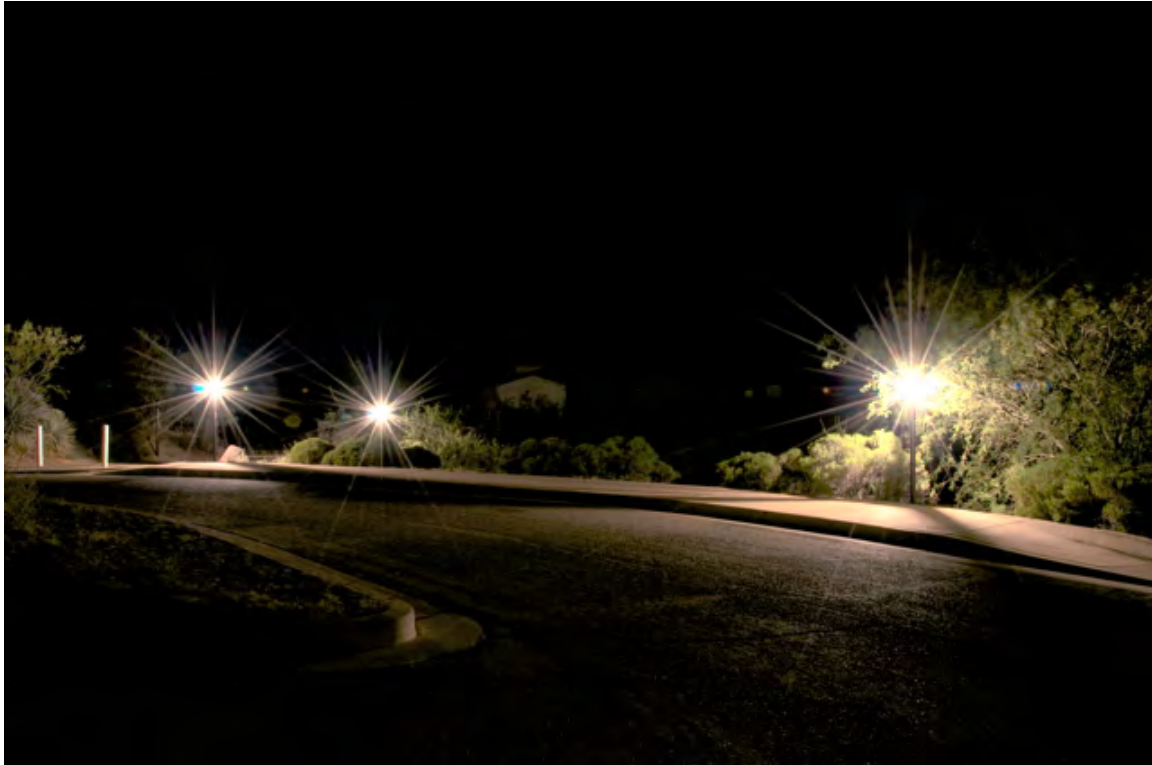
Figure 6.1 Kannally Ranch House parking lot lighting “before”
