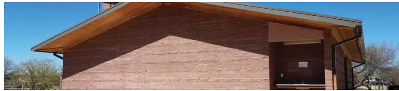
GROUP AREA: RESTROOM/SOWER BUILDING
