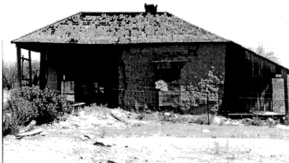
The last standing building associated with Fort McDowell, now demolished
