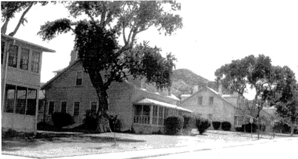
Some of the quarters for officers at Fort Huachuca
