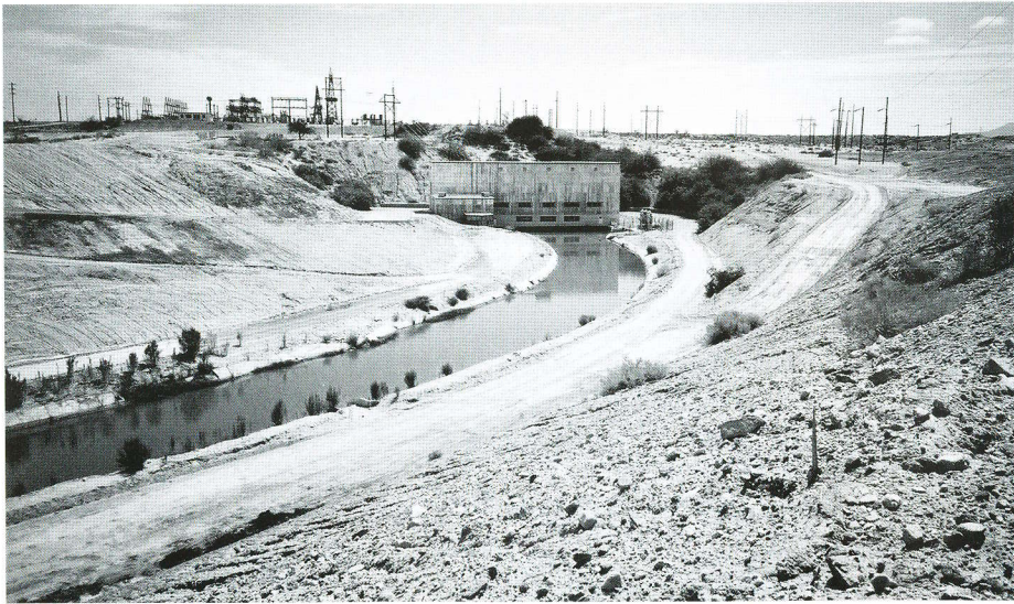
A Special Problem structure, represented by Lift Station No. 2 built in 1952 on the Bureau of Reclamation’s Wellton-Mohawk Project near Ligurta in Yuma County, lifts Colorado River water more than 50 feet to irrigated lands of the lower Gila River valley. Photograph by James Steely, SWCA.
