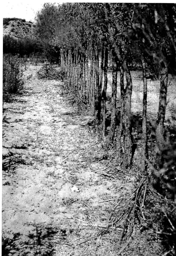
Figure 4.4. An example of a tree row diversion weir in the vicinity of the Río Sonora (photograph courtesy of Paul and Suzanne Fish).
