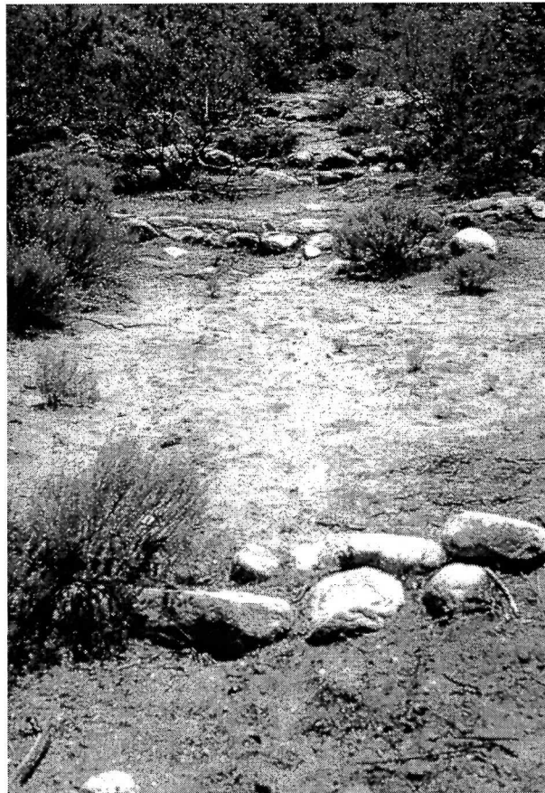
Figure 3.7. Check dams in the Goat Hill, Safford Valley area (photograph courtesy of Paul and Suzanne Fish).
