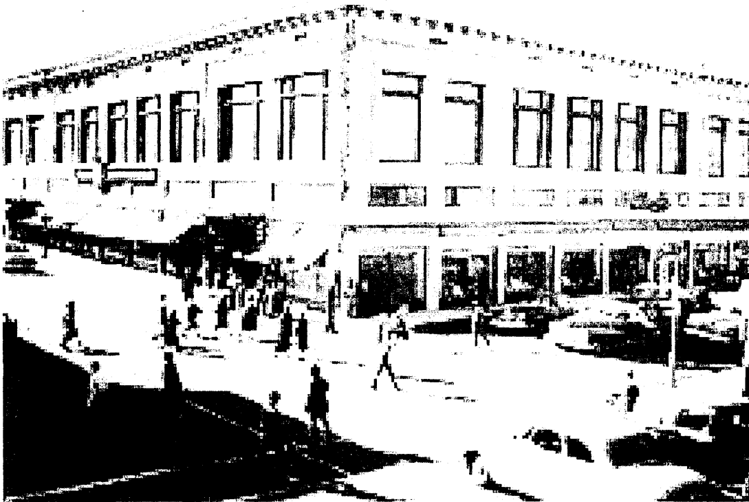
Photo 4-1. Steinfeld's Department Store at Stone and Pennington, n.d. (from Henry, Another Tucson , p. 123)
