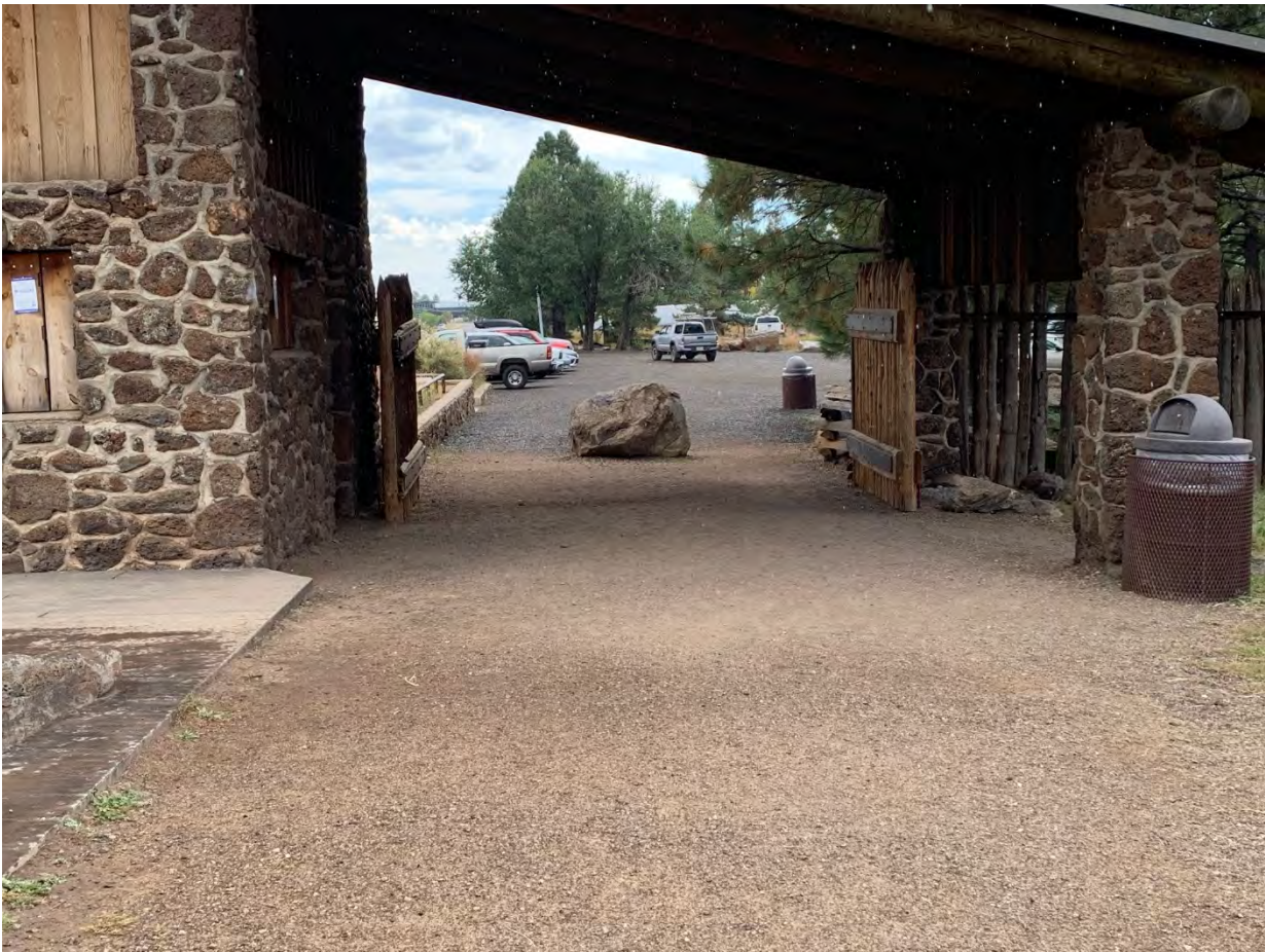
Looking through the entryway back to the parking lot
