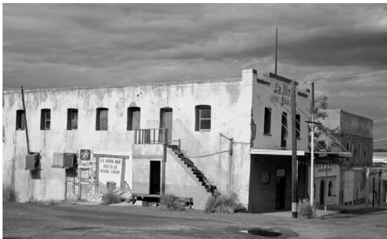
Small communities such as Superior (pictured above), contain numerous historic resources from their earliest days, which may be rehabilitated as part of their strategy to promote renewed economic activity.
