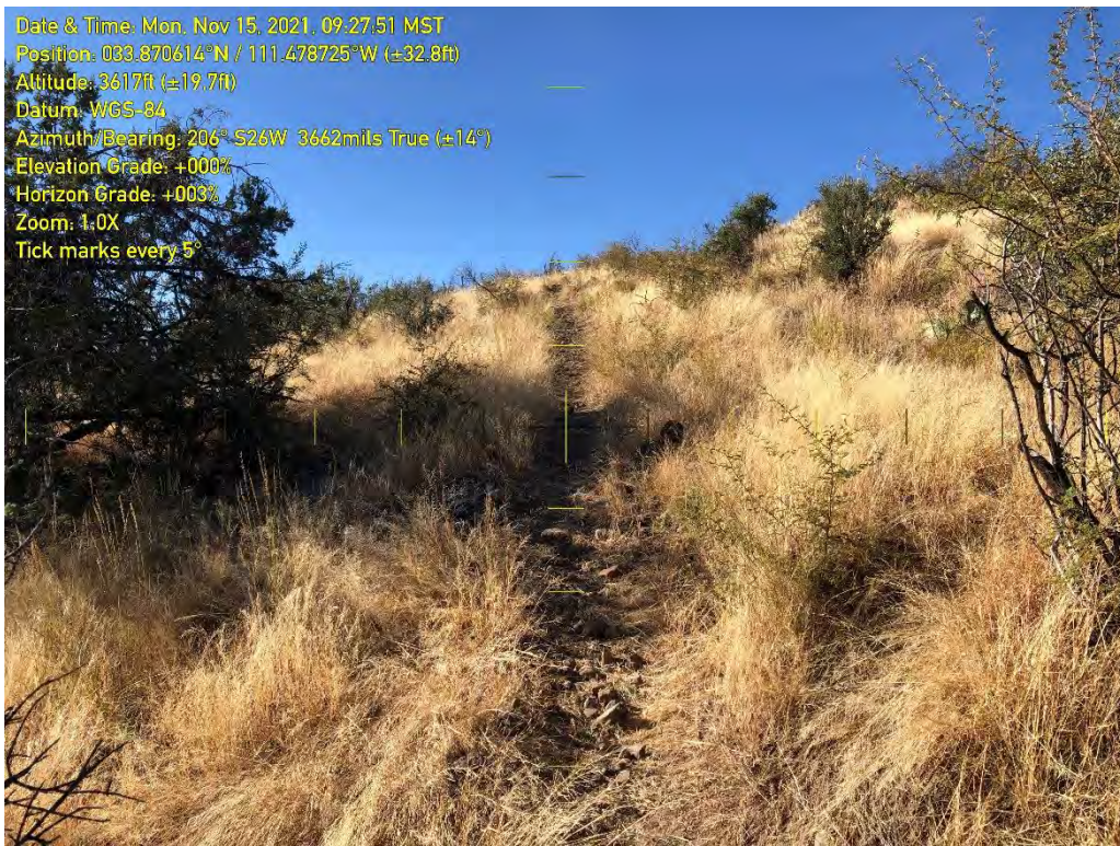
Steep, eroding climb near south end of the project. Project will realign around this hill.
